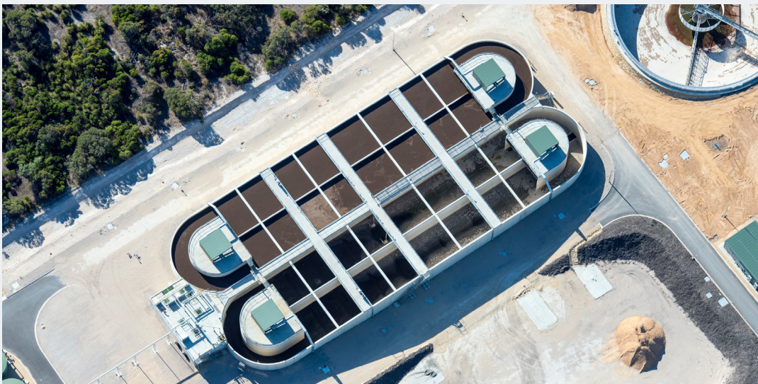
DBS Racetrack OXIDATION DITCH
